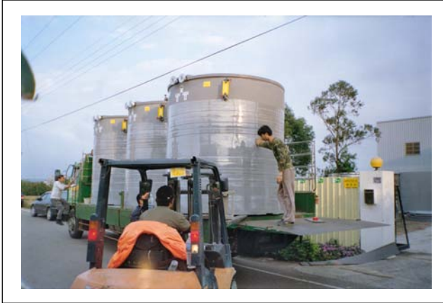
儲冰槽卡車運輸 Ice storage tanks transported by truck
