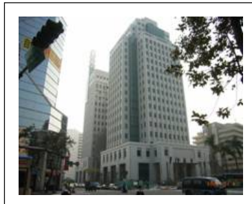
交通部仁愛大廈 Ren-ai Building, Ministry of Transportation And Communications Dyn-225 × 28 台 (sets)
