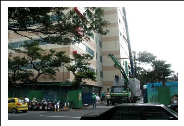
儲冰槽吊裝 Hanging the ice storage tank
